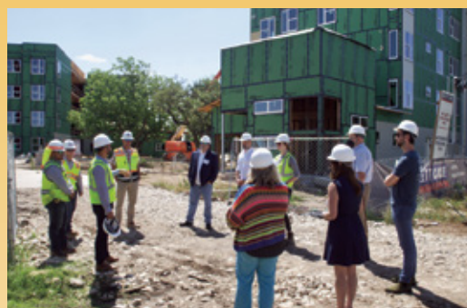
Event attendees tour construction of The Loretta
